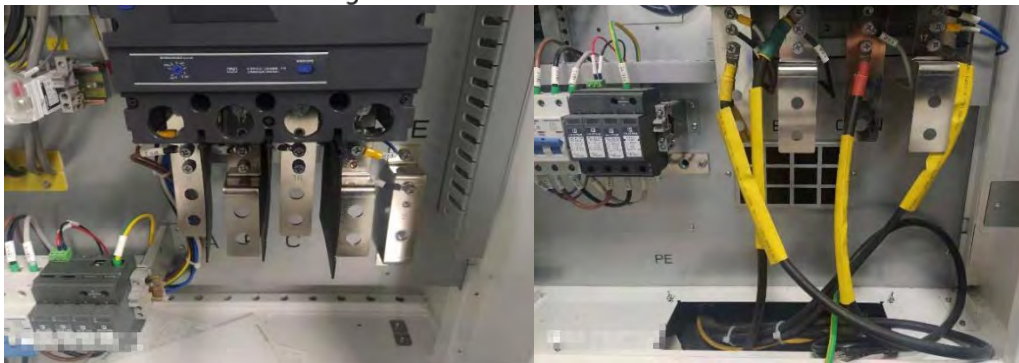
Figure 4-9 Position of PE
